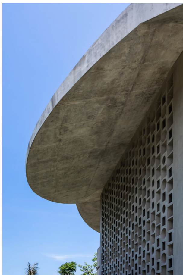
Ventilation block surface
