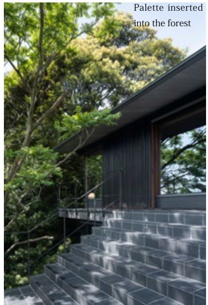
The sky space is on the right and the piano room is on the left. The floor height of the sky space is 1400mm lower than the second floor to match the slope of the site. The floor of the piano room, like the terrace, is finished with paver tiles, and when the sliding glass doors are opened, the interior and exterior are seamlessly connected. The height from the floor to the eaves is 2300mm.
